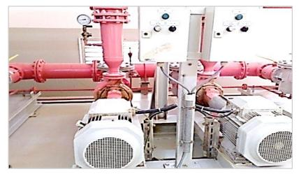
Figure 6. X5 location: Fuel forwarding pump unit (FFPU).
