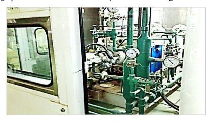
Figure 5. X4 location: High pressure feedwater pump (STU2).
